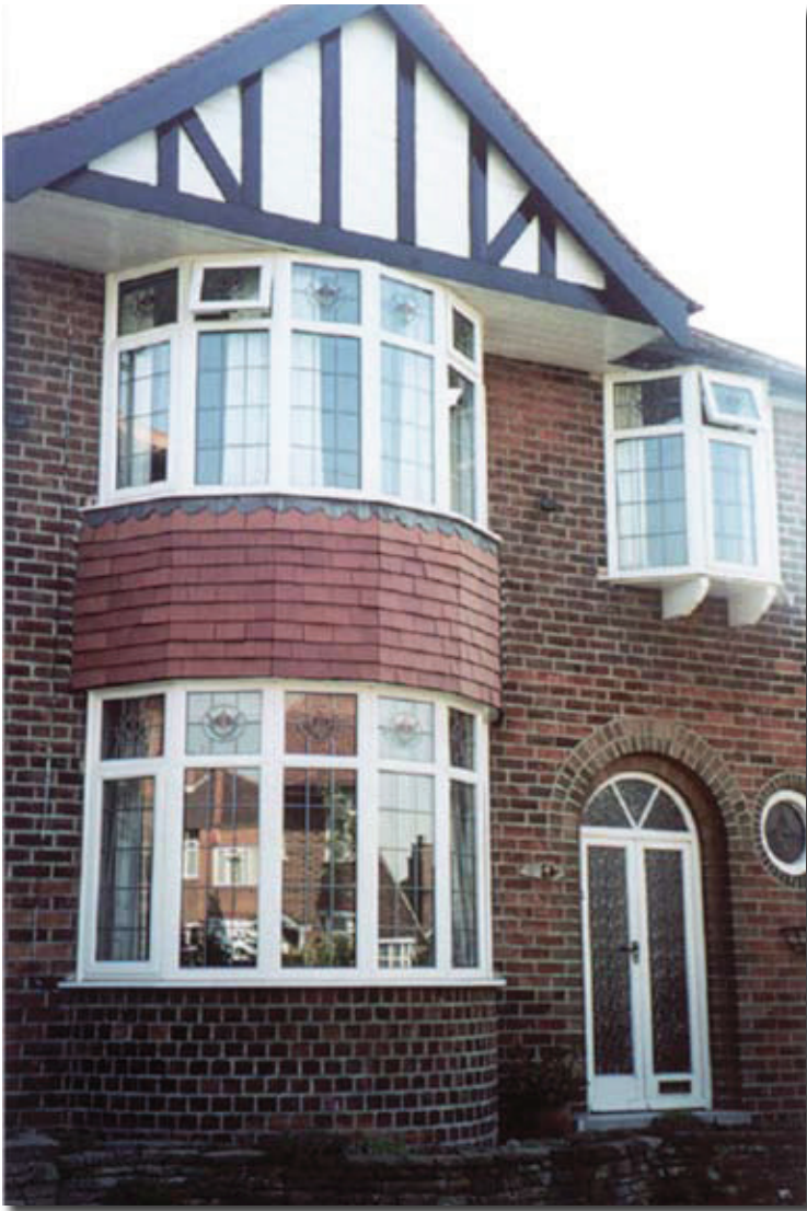
Bay windows can be easily and sensitively renewed.
